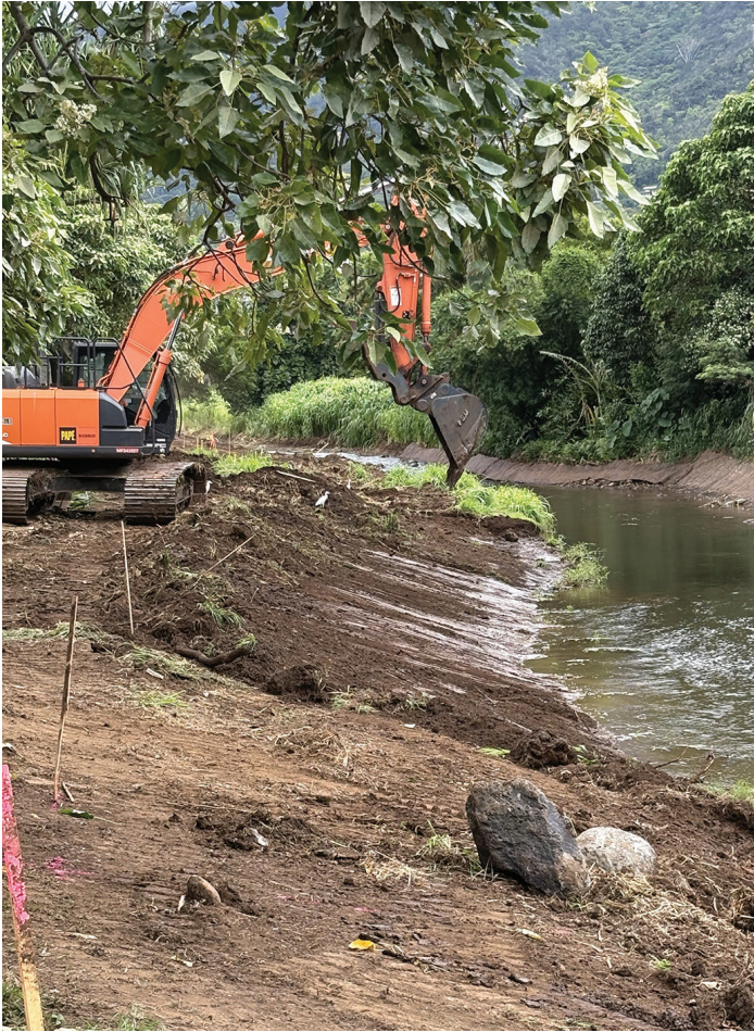
An excavator reshapes the bank of Mānoa Stream in August as crews begin the joint State and City flood mitigation work.
